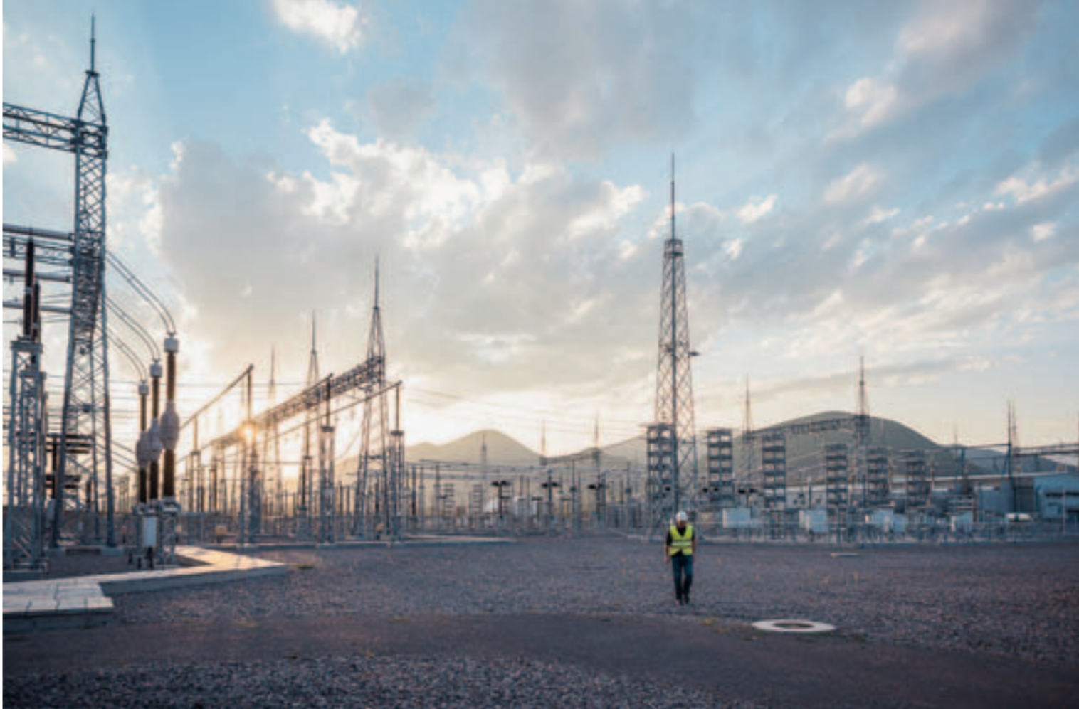
The Akhaltsikhe HVDC substation operates on two back-to-back links, each line of which is able to transmit 350 megawatts of power; the station can connect unsynchronized power from the Georgian 500-kilovolt system to Turkey's 400-kilovolt standard.
